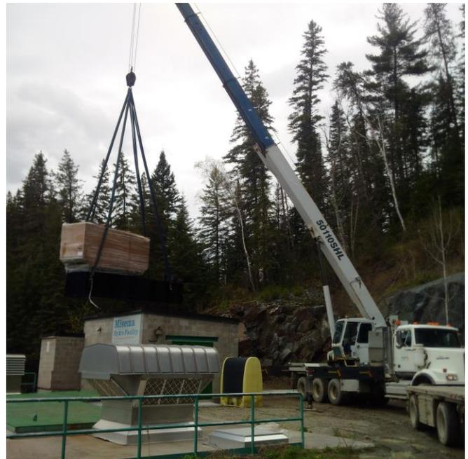
**Crane unloading and placing 125 kW genset**
