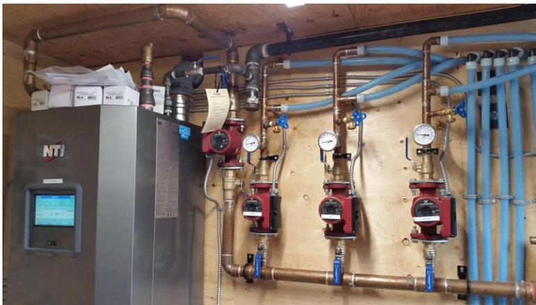
**Boiler and pumps for 3 heating zones in gate**
