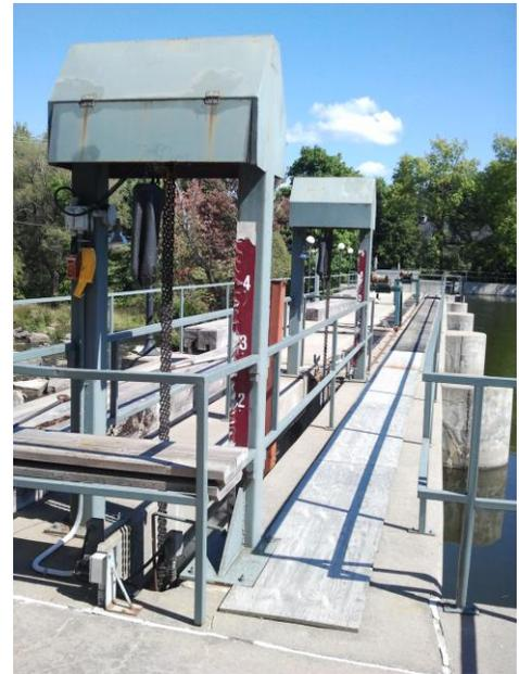
**These pictures show the original chain hoist system (right) and the small, wooden shack (left) housing the electrical. Note the two pendant controls on the hoist structure that operated each hoist independently.**
