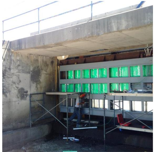
**Heating loops installed inside gate**
