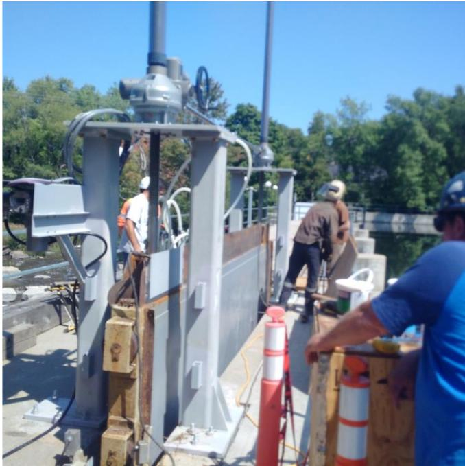
**Dual screw stem actuator and structure**
