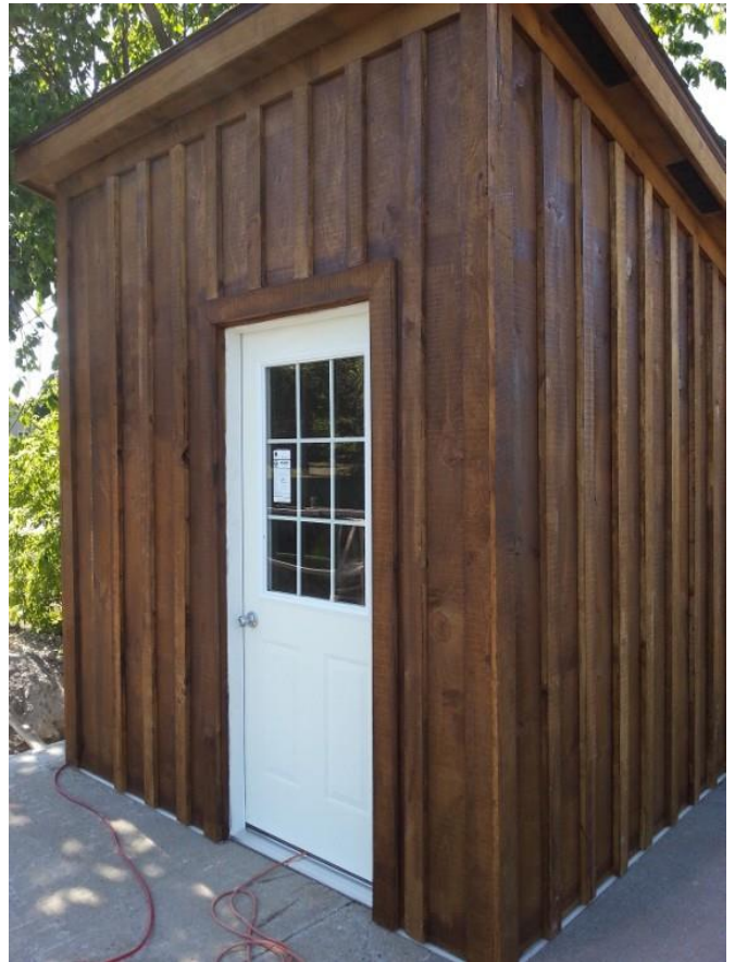
Outbuilding housing controls and boiler
