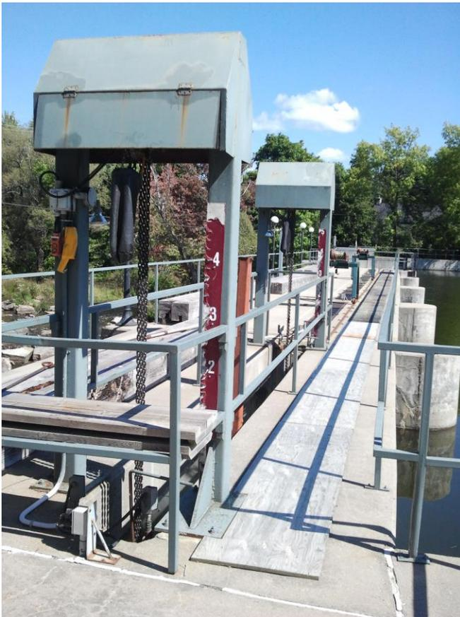
*These pictures show the original chain hoist system (left) and the small, wooden shack (below) housing the electrical. Note the two pendant controls on the hoist structure that operated each hoist independently.*
