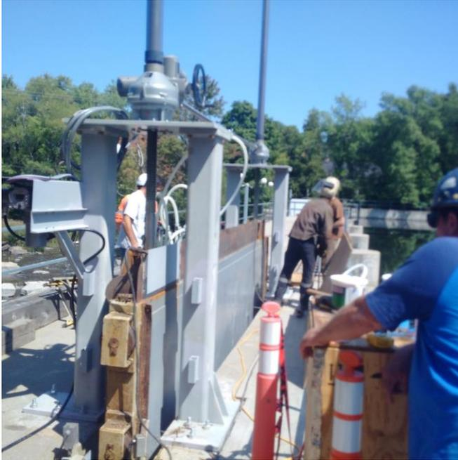
*Dual screw stem actuator and structure*
