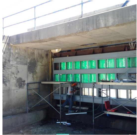
Heating loops installed inside gate
