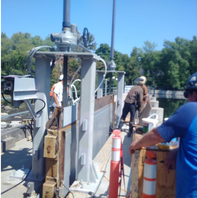
Dual screw stem actuator and structure
