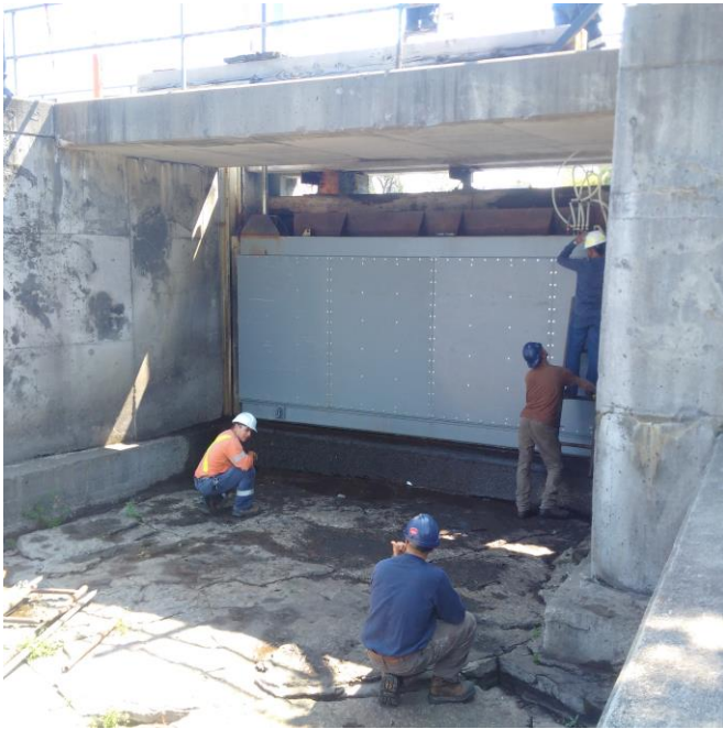
Sluice gate with new downstream skin
